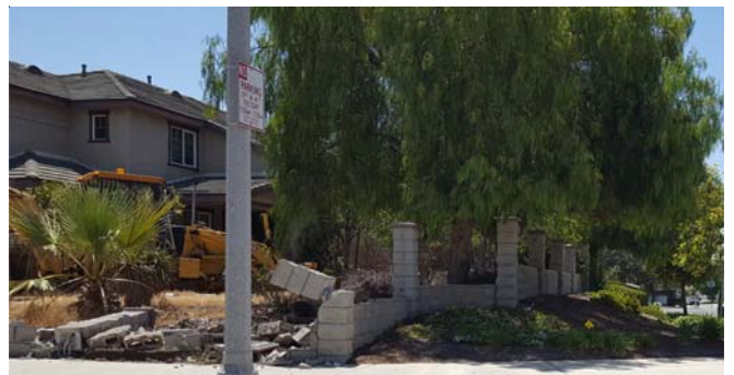
Association removal of wall
